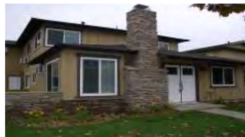
After Rehabilitation Improvements
