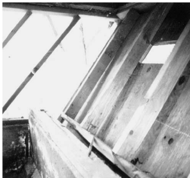
Figure 19 - This photograph shows an interior detail of a home similar to the one above, with substantial damage to a building with an unbraced tall wall.
