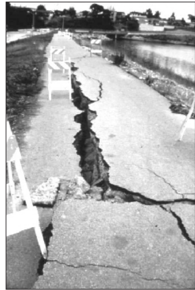
Figure 35 - Lateral Spreading, Loma Prieta Earthquake, October 17, 1989. Lateral spreading damaged levee road along the San Lorenzo River.
