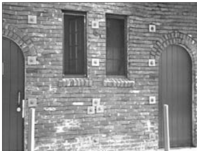
Figure 24 - Bolting of unreinforced masonry wall to steel frame on the inside.
