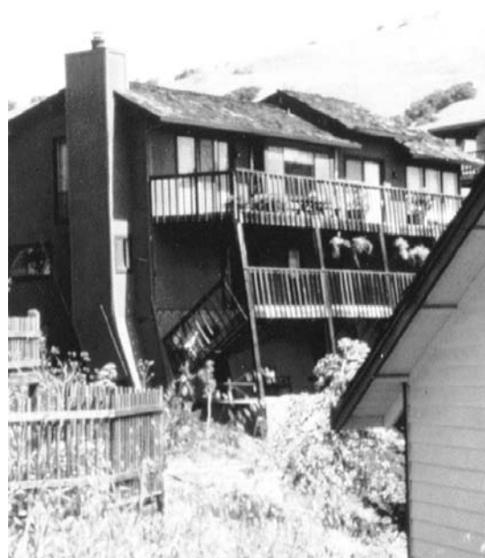
Figure 18 - This hillside home was built on an unbraced tall wall that failed.
