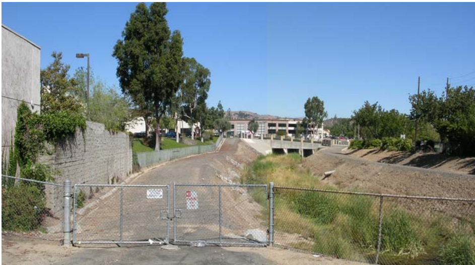
Loftus Channel, view north, between Imperial Highway Associated Road bridge
